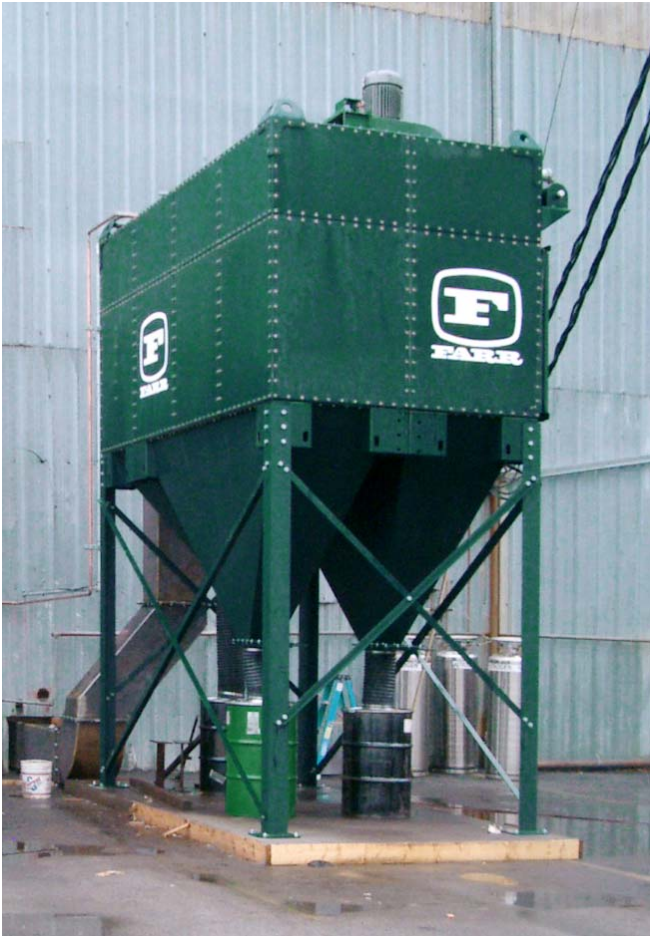
Farr Gold Series GS24 installed at Chatham Steel on a plasma cutting table application.
