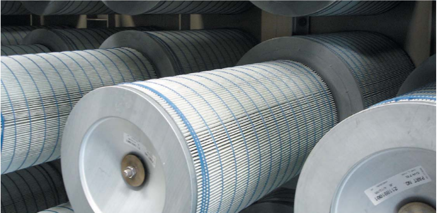
HemiPleat retrofit into a horizontal gas turbine intake filter.
