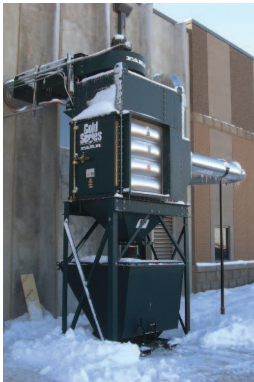
Collector serving wood form shop is equipped with an explosion vent and an underground ducting and automated control system.
