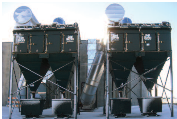
Gold Series® GS48 dust collectors serve the sandblasting bays.
