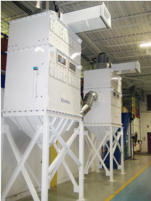
*Type "B" Central Wet Collectors - Drain Valve Dust Removal*
