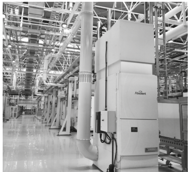
One filter unit - several machines. Installation at Volvo Zhangjiakou, A•mist 80TF
